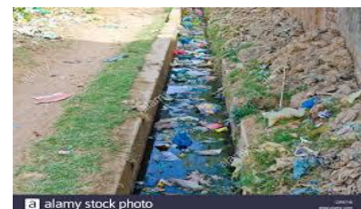
Fig.2. solid waste in drains
